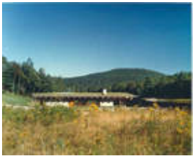
Tennis House, Washington, Connecticut Gray Organschi Architecture, New Haven, Connecticut
