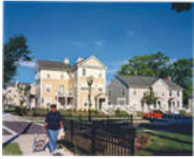
Monterey Place, Hope VI, New Haven, Connecticut Fletcher Thompson Inc., Shelton, Connecticut
