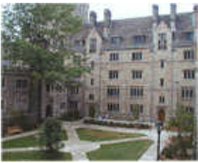
Branford and Saybrook Colleges Renovations, Yale University, New Haven, Connecticut Perry Dean Rogers and Partners Architects, Boston, MA
