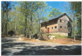
Old Usquepaug Residence, Richmond, RI Lindsay Suter, Architect, North Branford, Connecticut
