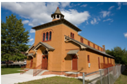
Recital Hall at Betsy Ross School, New Haven, CT Barkin Associates Architects, P.C./JCJ Architecture, Hartford, CT
